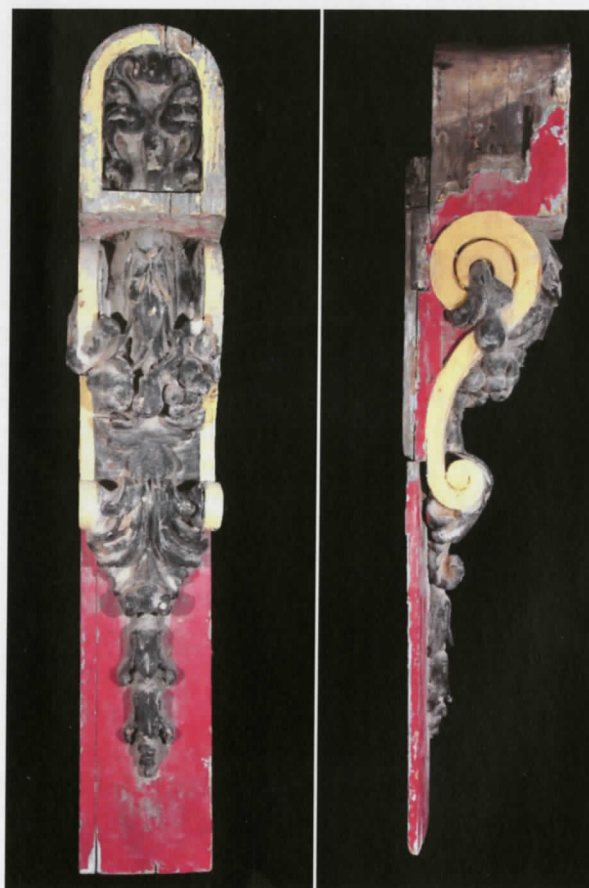
Fig 3. Front and side of main decorative console. The wooden construction has many oblong splits. The paint layer has many losses and extensively flakes unveiling previous paint schemes.
